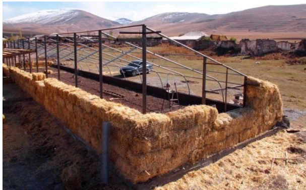
Picture 1. PSG in Kut village, Gegharkunik region. Picture taken during construction, 2013.
