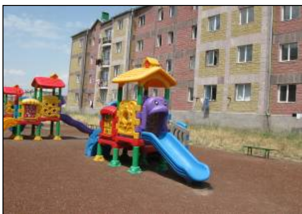
A multi-apartment inhabited residential building in Mush-2 district
