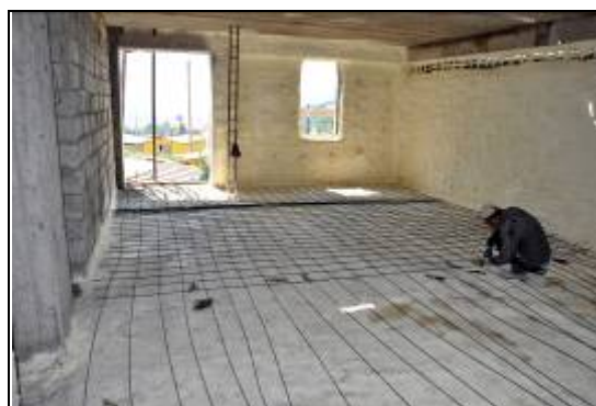
Insulation of the floors
