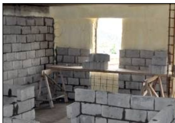
Covering of the wall insulation with blocks
