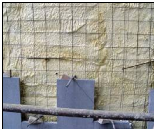
Thermal insulation of the external walls
