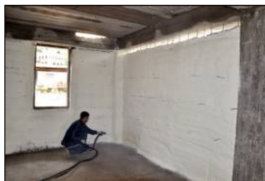
Insulation of the walls
